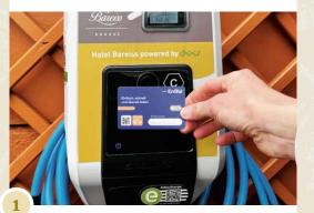
Hold the charging card up to the RFID reader or scan the QR code on the wallbox with your smartphone camera.
